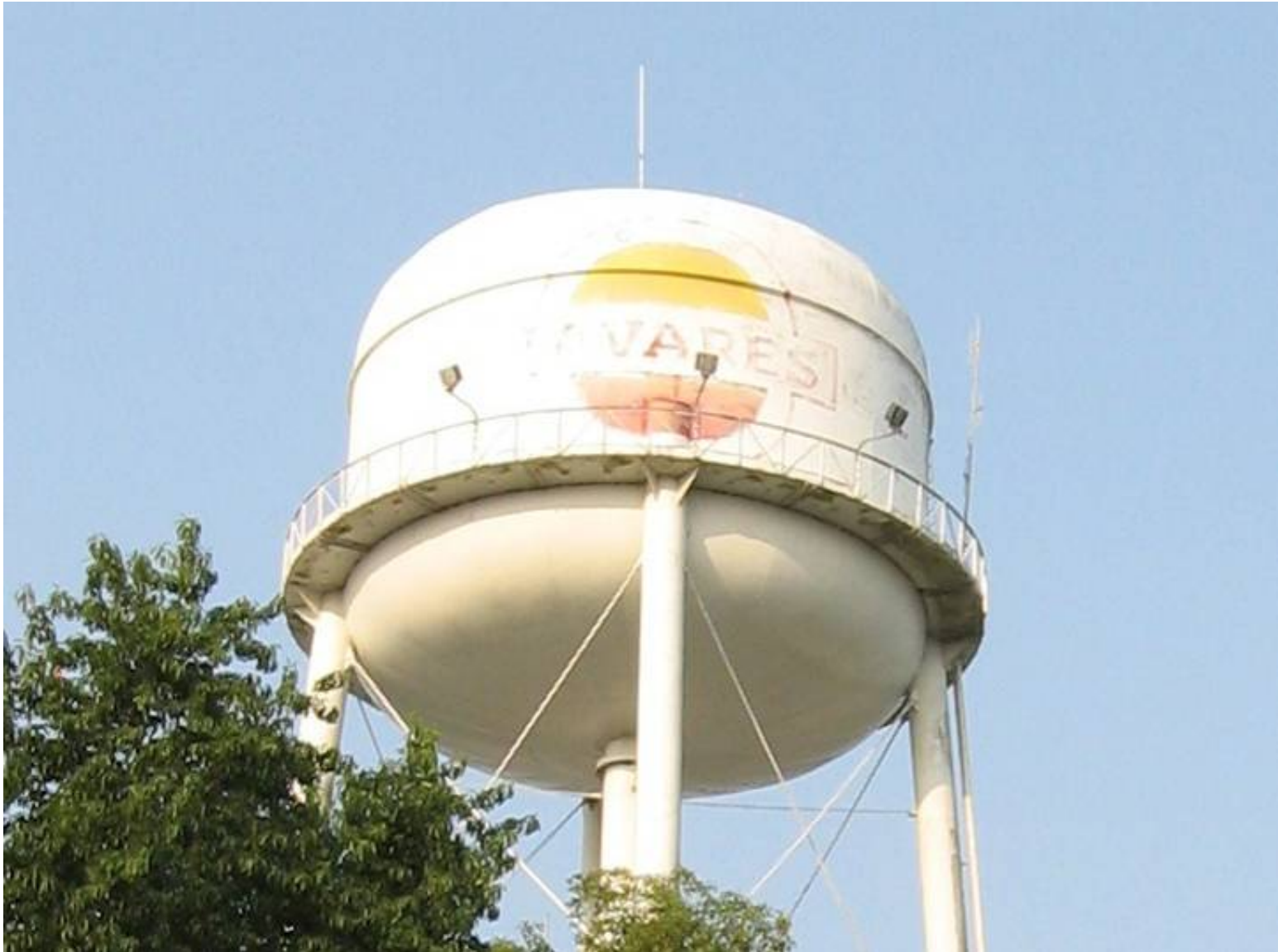
200,000 Gallon Water Tower
