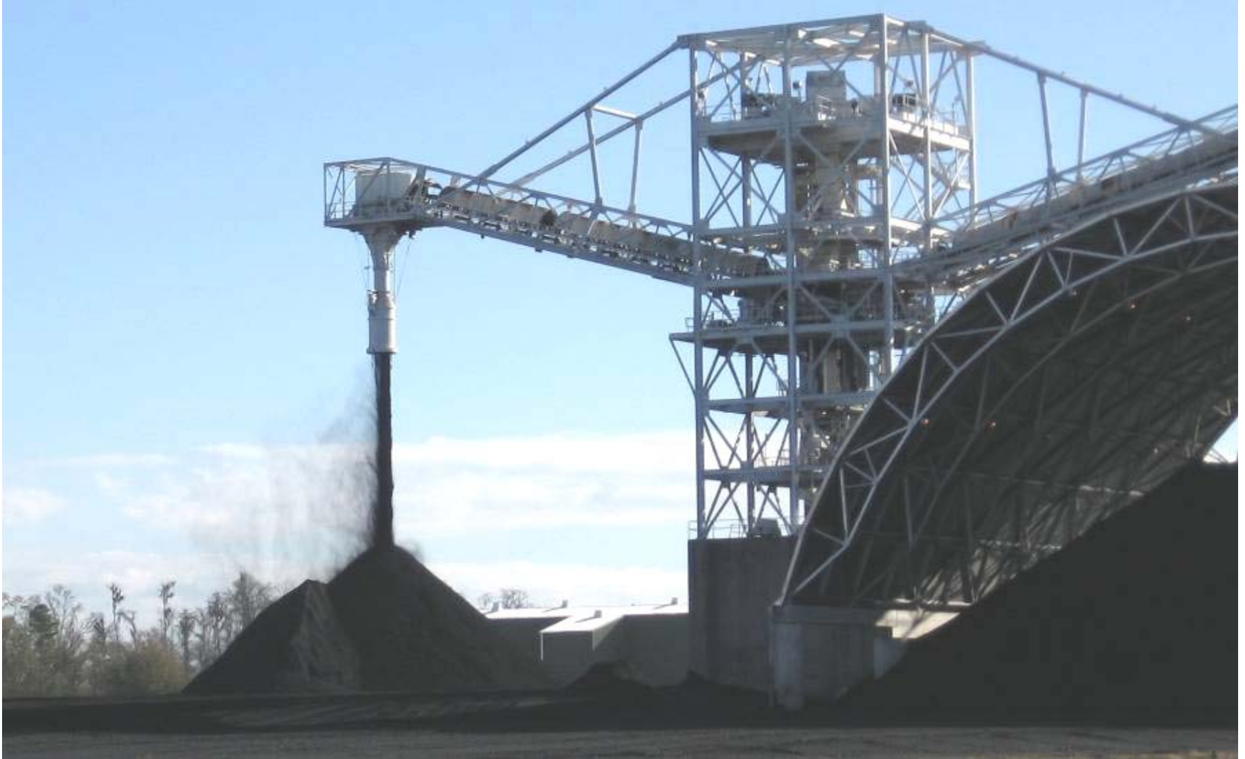
Unloading Coal Hoppers
